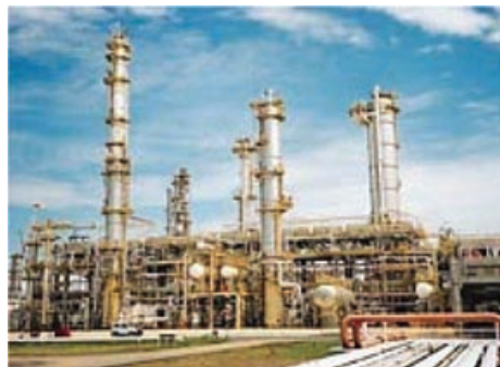
Fluid heating in a petroleum process heater.
